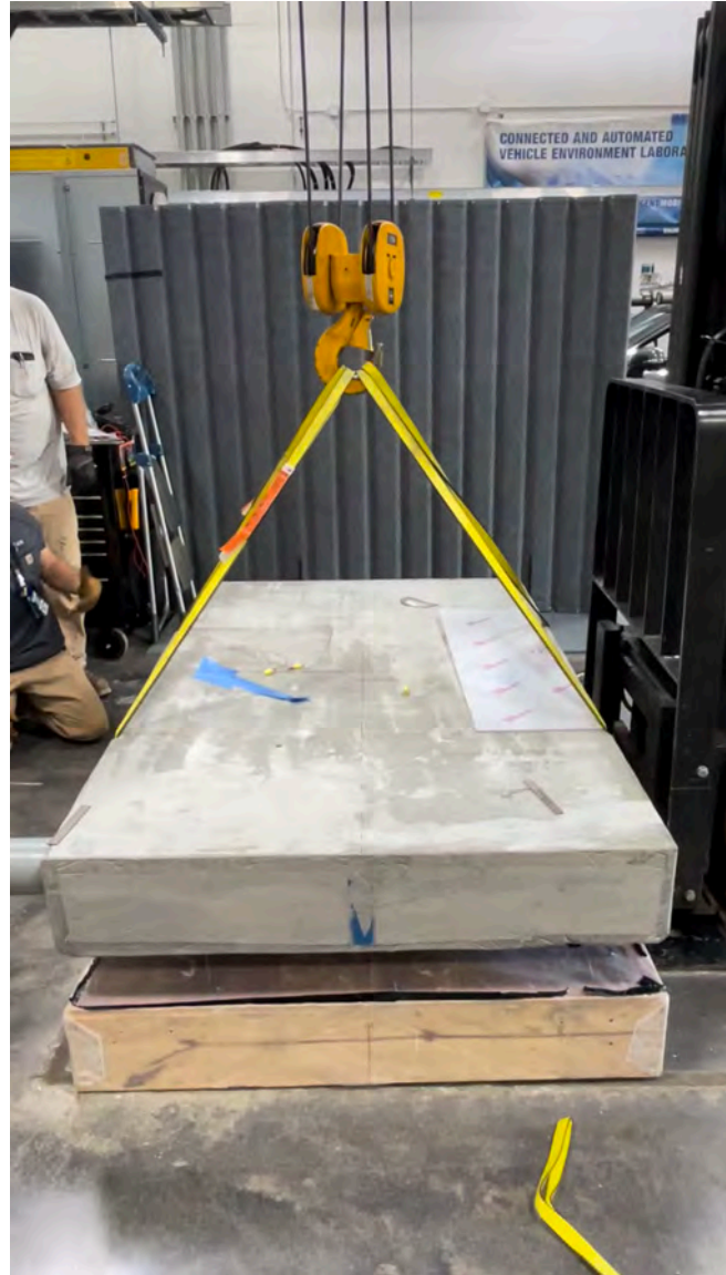
200 kW DWPT transmitter set in precast Master flow 648 Epoxy Resin Grout
