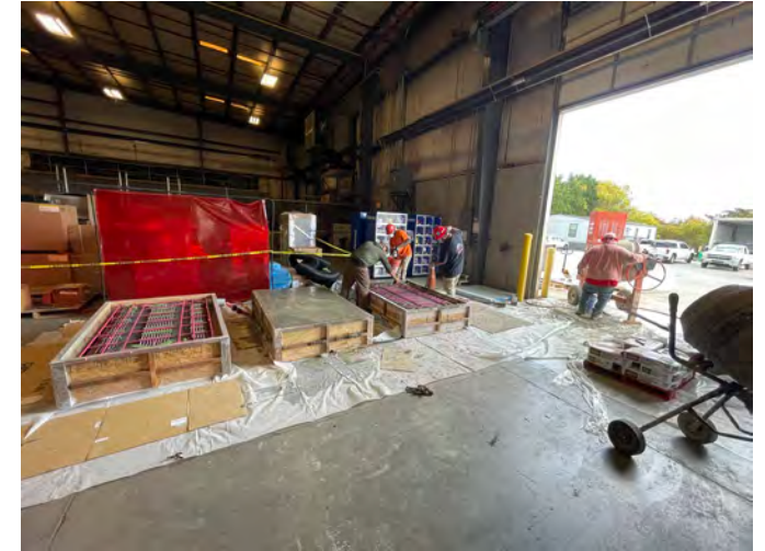
Coils with fiber glass re-enforcement being concretized
